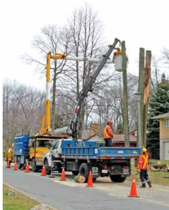
Aerial device and crane
